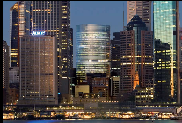
1 Bligh Street - commercial tower, under construction (with Ingenhoven Architects)
